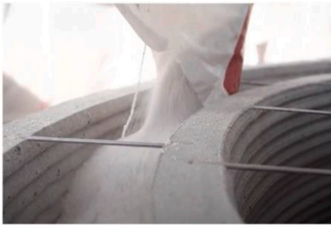
Fig. 2. Addition of insulation material within printed wall (Palazzo, 2025).
